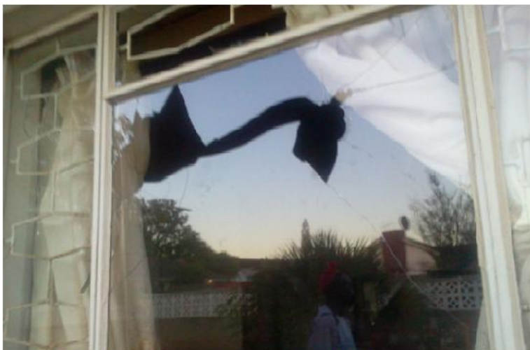
Broken window at Dorcas Sibanda's house
